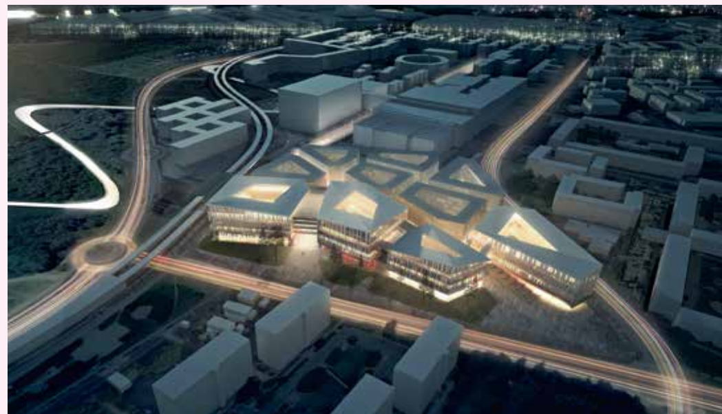
FOTO: HENNING LARSEN ARCHITECTS
